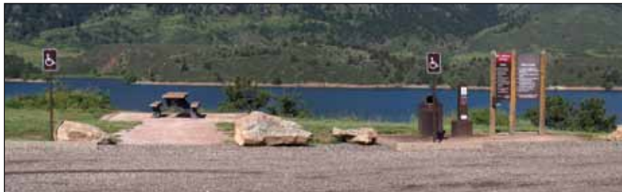
ADA upgrades on the east side of Horsetooth Reservoir Photo: Steve McCorkel
